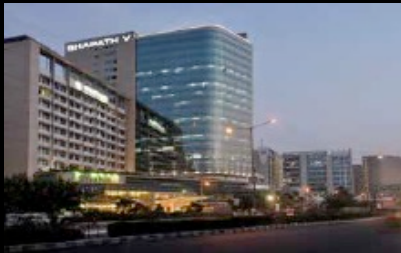
OFFICES & INDIAN SALES (AHMEDABAD, INDIA)
